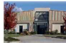
The GTPDD office is centrally located in Oktibbeha County in the Starkville Industrial Park
